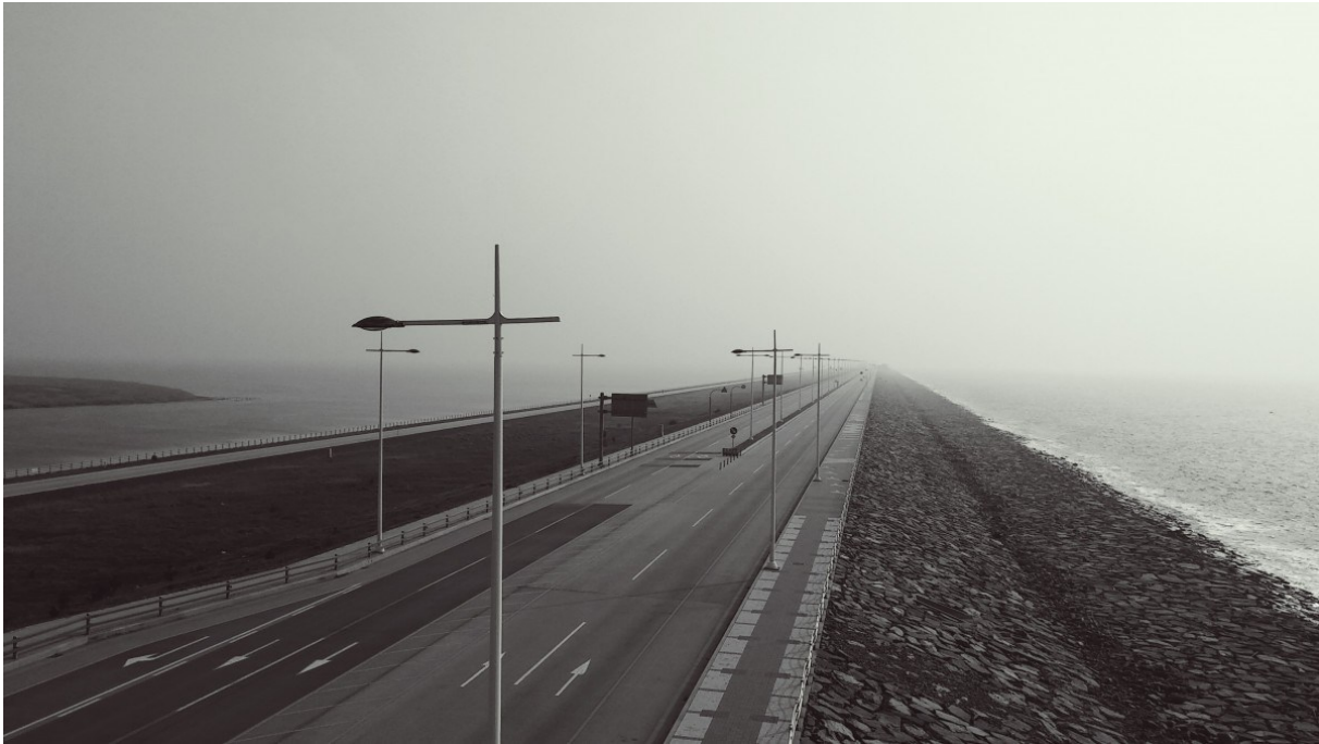
Image 1. Using a single means for two or more goals: a dyke and a road (image: Pxhere)
